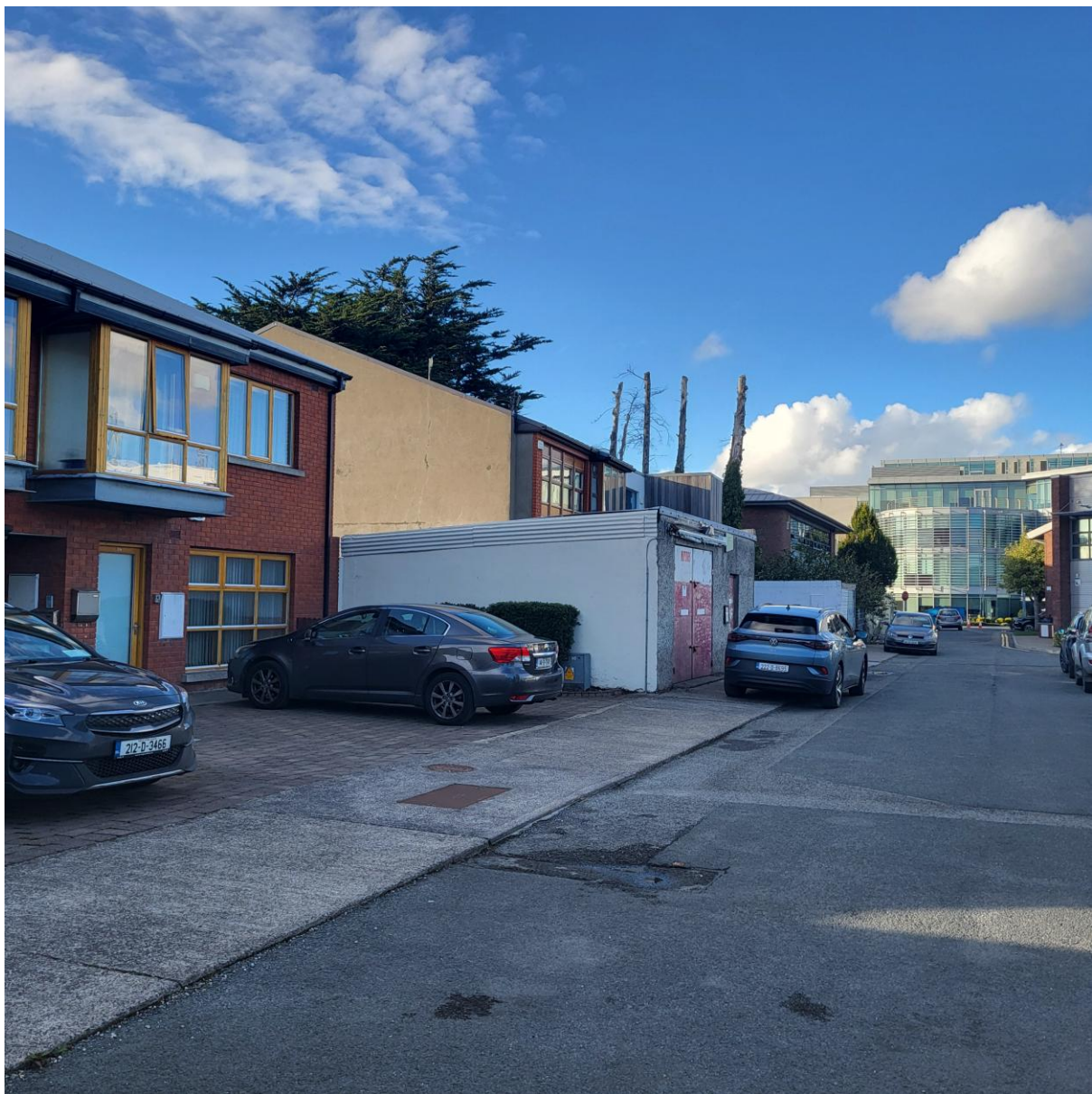
Current building projecting out from building line, proposed development will be similar.
